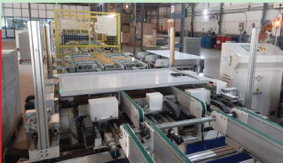
JUNCTION BOX INSTALLATION
